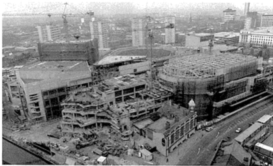
Under construction: Birmingham's £121 million International Conference Centre - opening in 1991.
